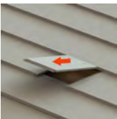
1. Remove the tile and locate the rafter.
