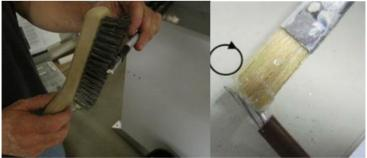
Figure 2.39 - Preparing Aluminum Wires Prior to Connecting
